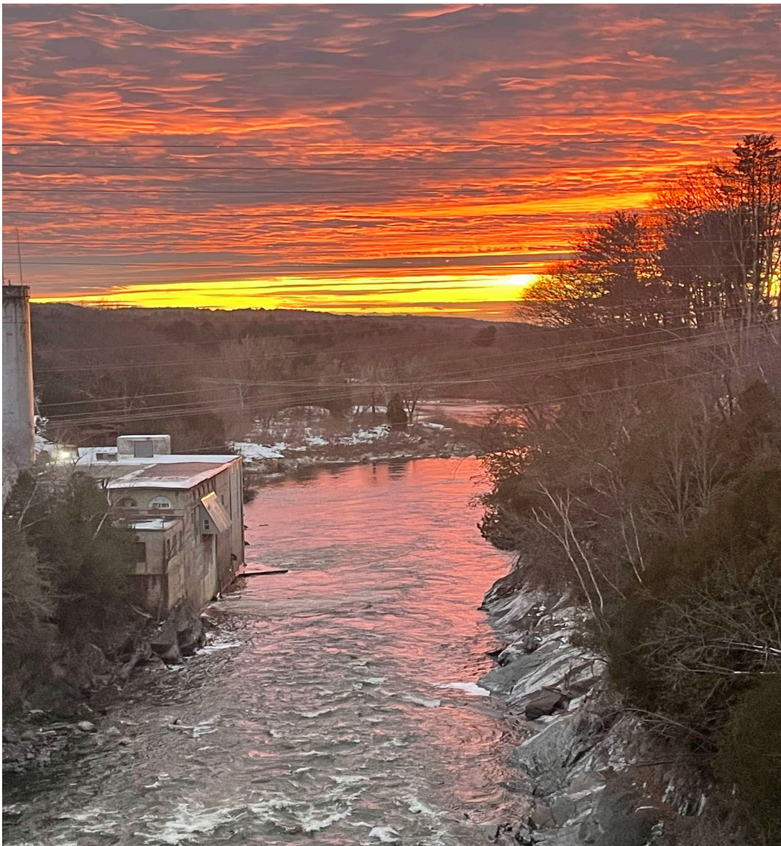
PHOTO CREDIT DAVID PRATT SUNSET AT ORMAN CROFT GENERATING FACILITY
