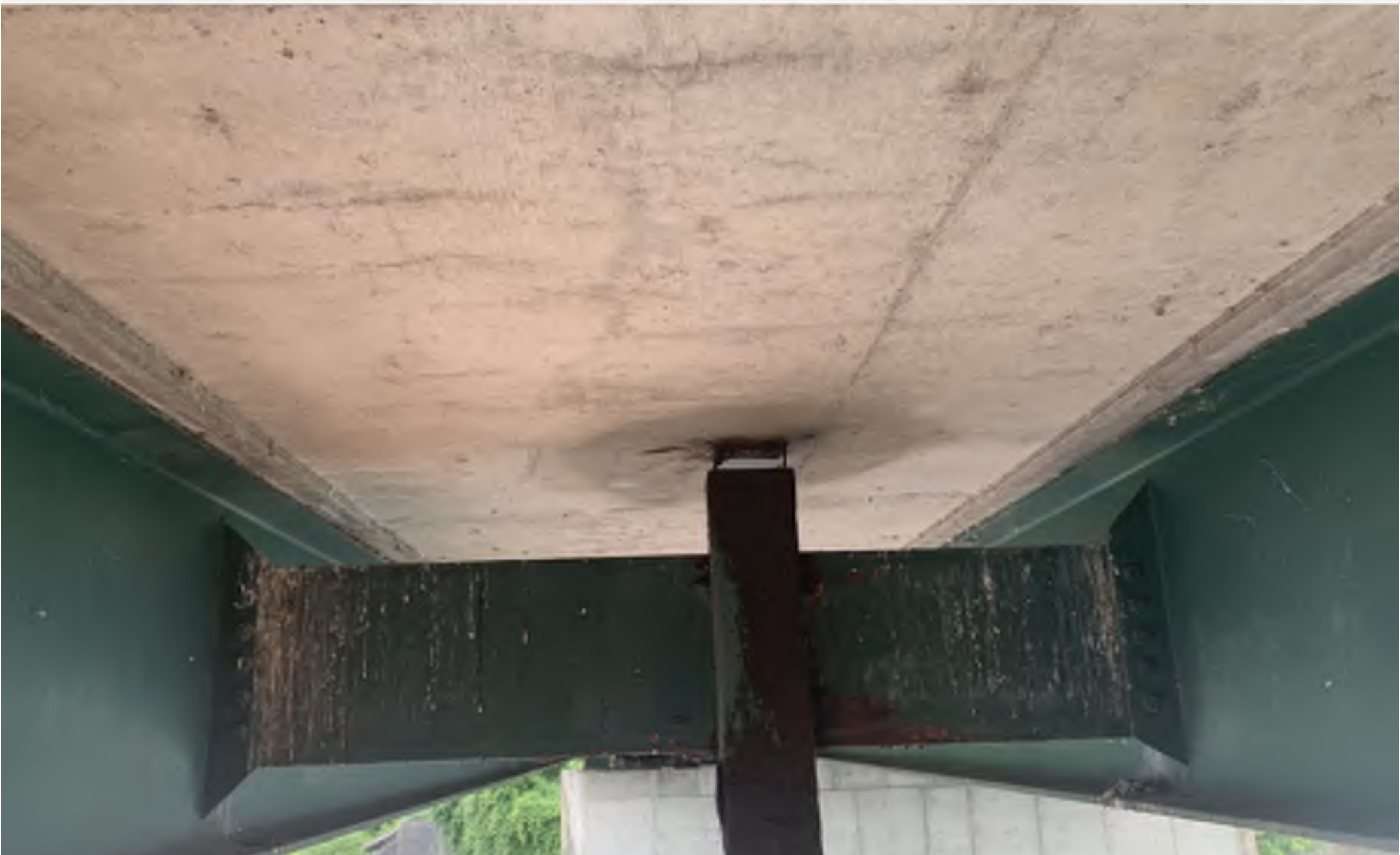
Typical Deck Drain
